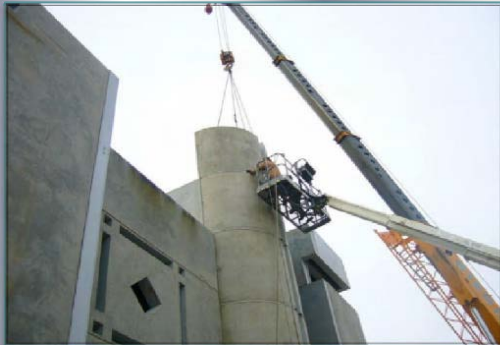
Installation of the last (curved) panel into place which brings to completion the overall assembly of the HCD Technology Center.
