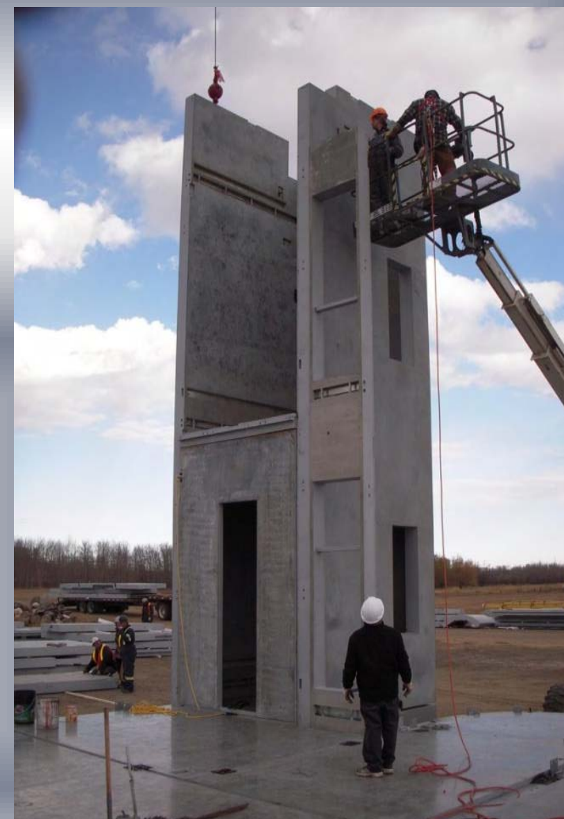
(left) Adding internal walls during the erection process, acted as lateral supports for the approx. 40' exterior wall panels to be erected. There was no need for any traditional heavy bracing.
