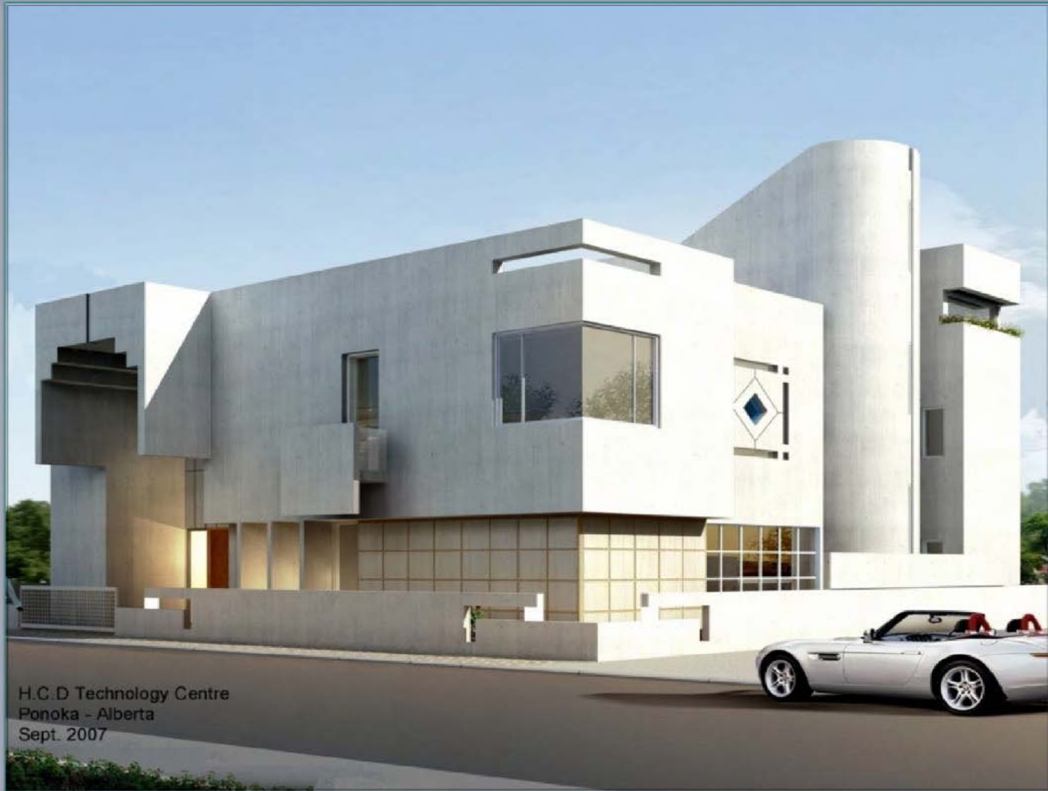
PERSPECTIVE OF MAIN ENTRANCE WITH UNIQUE SEAMLESS JOINTS & CONNECTIONS UNLIKE ANY PRE-MANUFACTURED PANELIZED ELEMENTS WHETHER MODULAR OR NOT.
