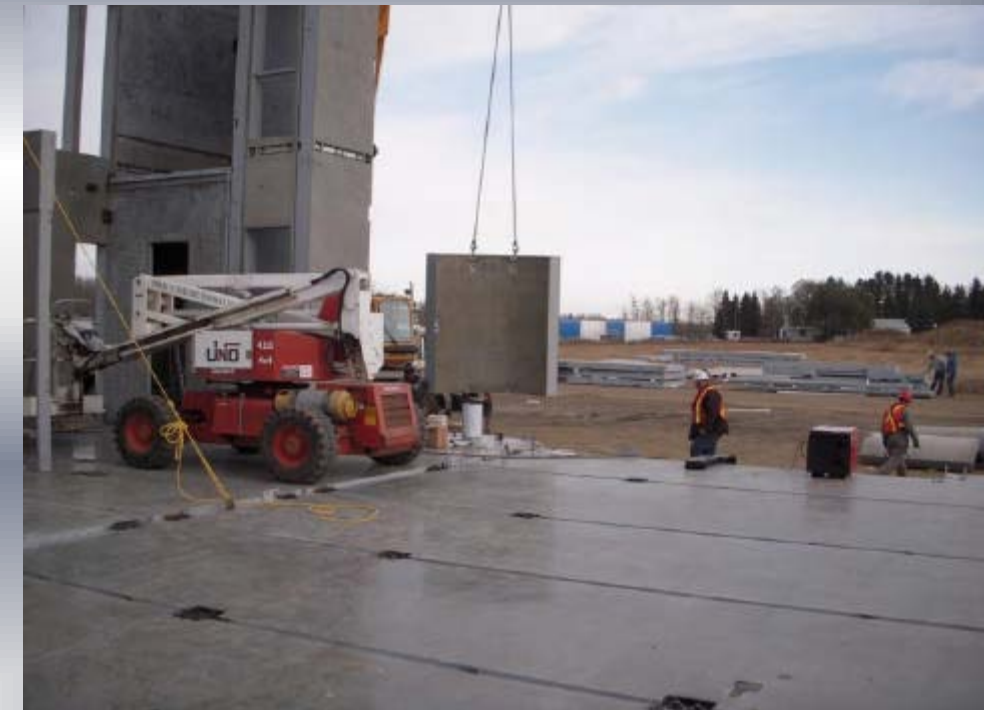
Assembly of first curved wall for the staircase.
