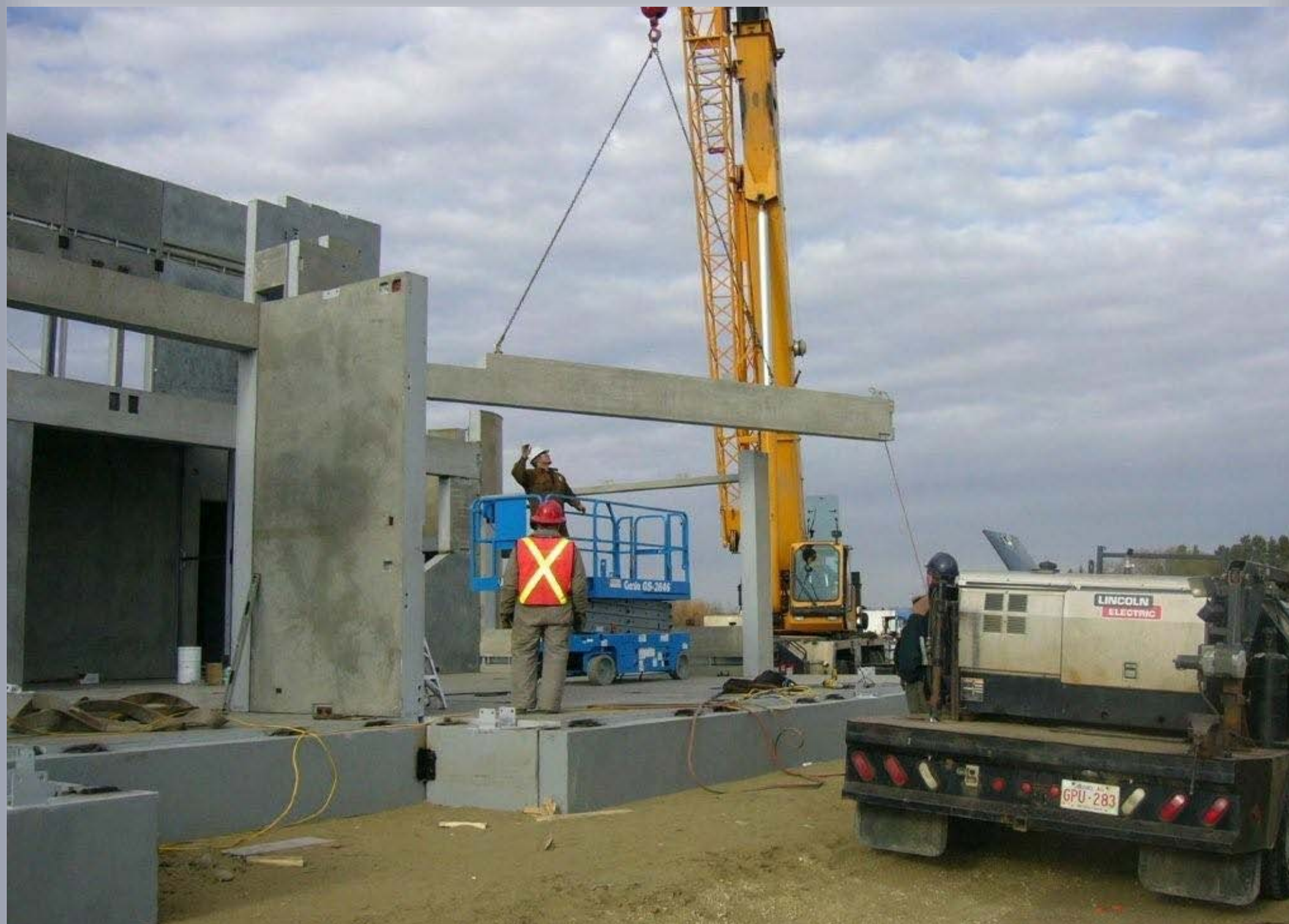
Installing an IHI beam into place.
