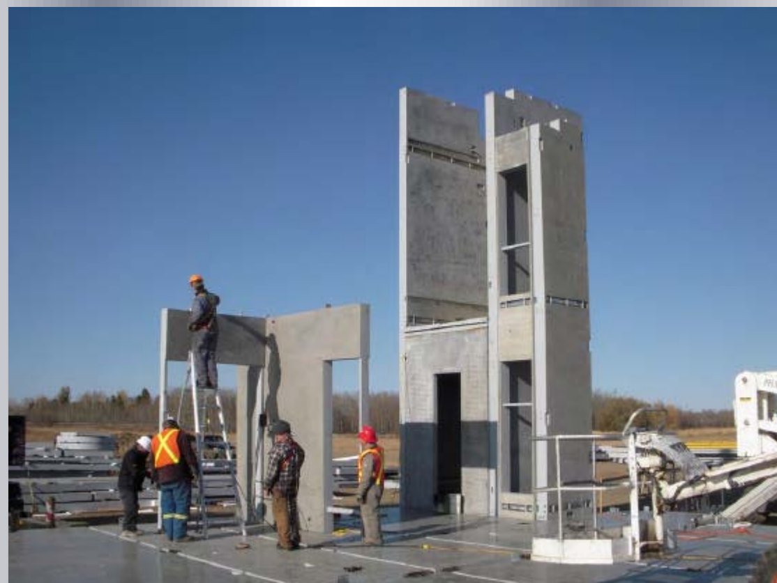
(left) Adding internal walls during the erection process, acted as lateral supports for the approx. 40' exterior wall panels to be erected. There was no need for any traditional heavy bracing.
