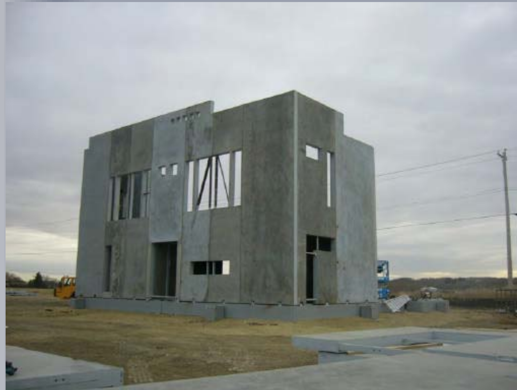
View from the South-West corner – rear entrance to the Technology Center . All temporary bracings within the window or door openings were knocked off after erecting the whole building.
