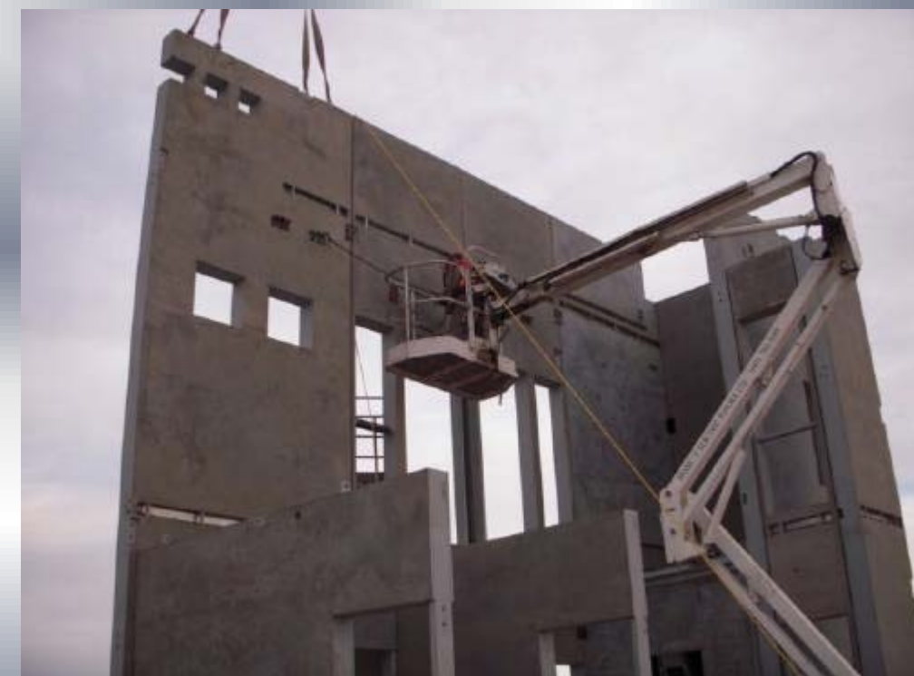
No bracing and/or scaffolding is required. All panels are uniquely architecturally and structurally integrated to each other.
