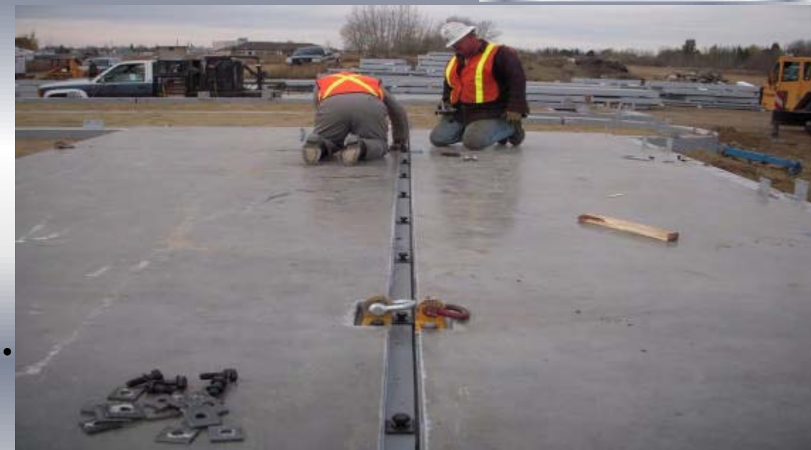
Perfectly smooth high-strength concrete panels connected through an open channel which can be easily used to pass extra MEP services if needed prior to filling with plaster.
