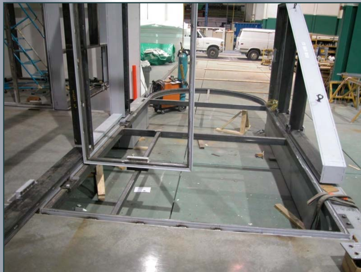
INTERNAL VIEW OF THE STAIRCASE AND ITS CURVED LANDING.
