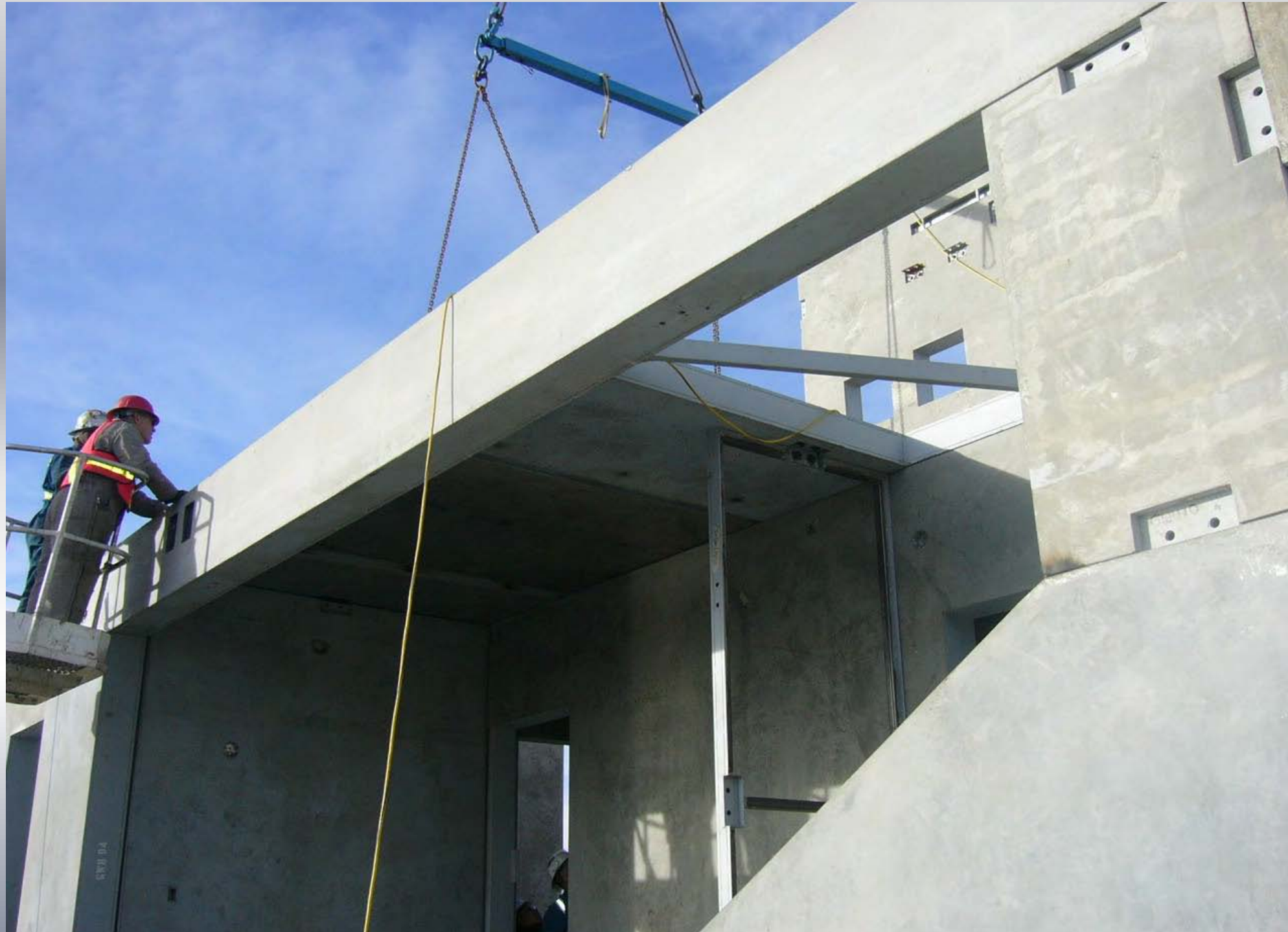
Assembly of second floor slab.
