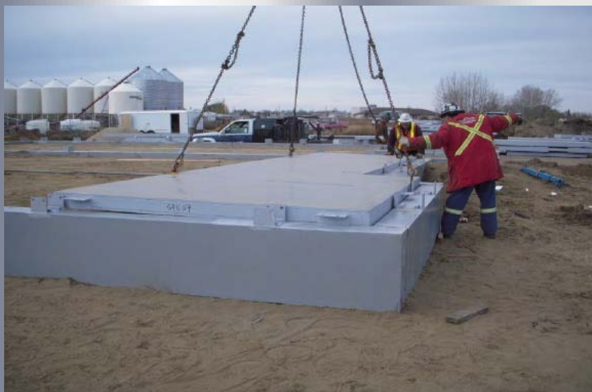
The IHI ground panel fits perfectly with the insulated foundation panels.
