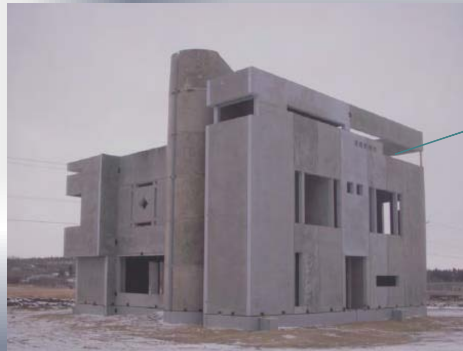
View from the South-West corner – rear entrance to the Technology Center . All temporary bracings within the window or door openings were knocked off after erecting the whole building.
