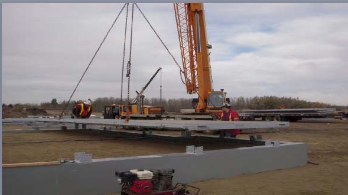
This picture shows a 30 ft. insulated ground insulated slab (6 inches thick) spanning with no deflection. A unique feature for IHI due to the high strength to weight ratio.
