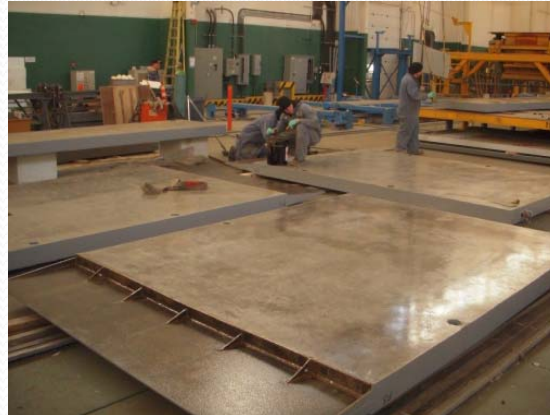
FINE FINISHING OF THE 12,000 PSI CONCRETE IHI PANEL
