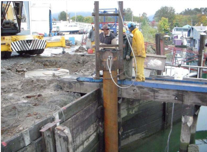
DRIVING PILES TO OCEAN BED
