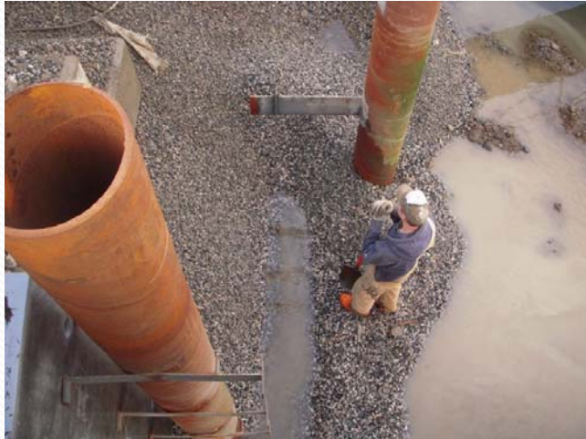
INSTALLATION OF STEEL PILES WITH SPECIAL WELDED BRACKETS, THIN AND ADJUSTABLE IHI BRACKETS TO CONNECT THE IHI PANELIZED PLATES.
