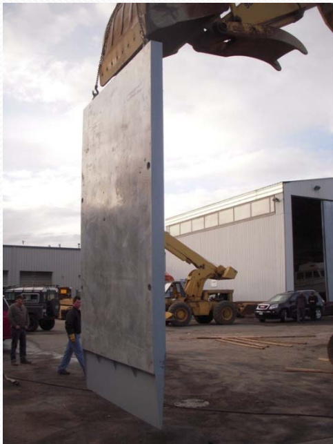
DUE TO THE FLEXIBILITY OF THE IHI SYSTEM, A BACKHOE WAS UTILIZED ON SITE TO INSTALL THE PANELS.
