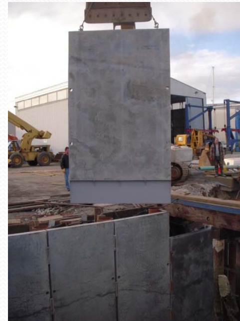
DUE TO THE FLEXIBILITY OF THE IHI SYSTEM, A BACKHOE WAS UTILIZED ON SITE TO INSTALL THE PANELS.
