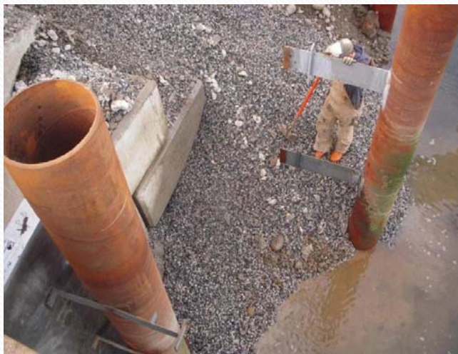
INSTALLATION OF STEEL PILES WITH SPECIAL WELDED BRACKETS, THIN AND ADJUSTABLE IHI BRACKETS TO CONNECT THE IHI PANELIZED PLATES.
