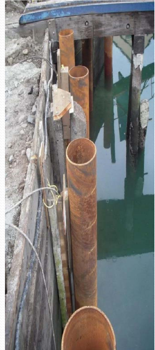
INSTALLATION OF STEEL PILES WITH SPECIAL WELDED BRACKETS, THIN AND ADJUSTABLE IHI BRACKETS TO CONNECT THE IHI PANELIZED PLATES.
