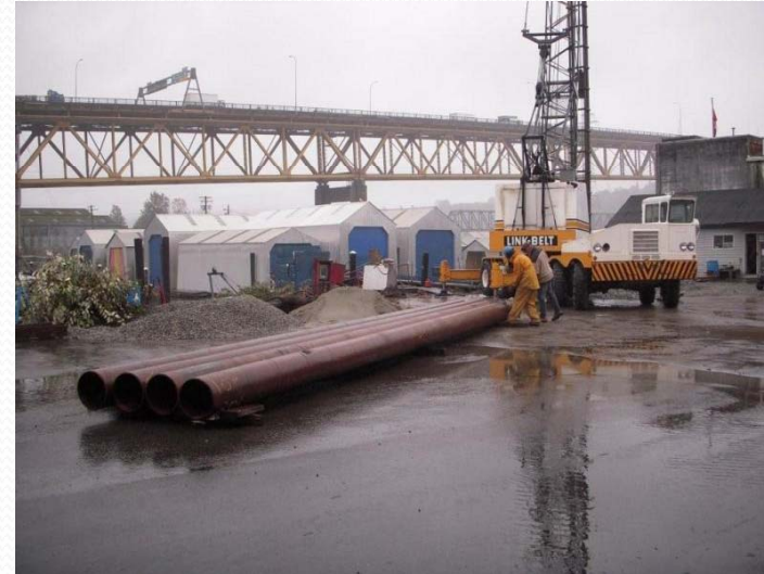
ARRIVAL OF STEEL PILES TO SITE
