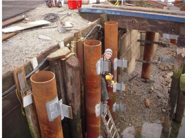
INSTALLATION OF STEEL PILES WITH SPECIAL WELDED BRACKETS, THIN AND ADJUSTABLE IHI BRACKETS TO CONNECT THE IHI PANELIZED PLATES.
