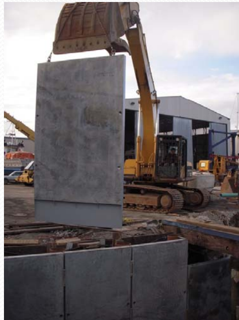
DUE TO THE FLEXIBILITY OF THE IHI SYSTEM, A BACKHOE WAS UTILIZED ON SITE TO INSTALL THE PANELS.
